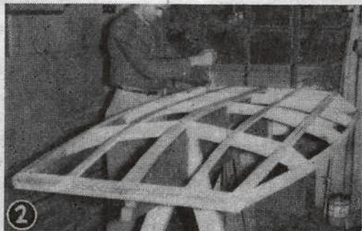
Bow view of framework on the building form.
