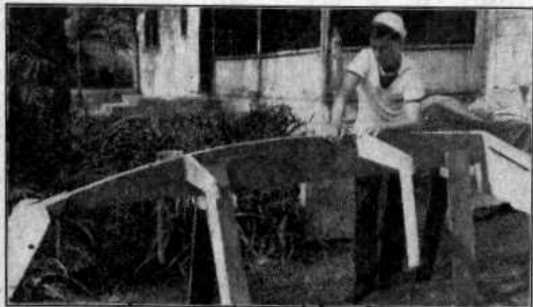
Putting the mould frames into place.
