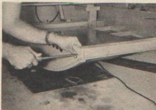
SCREWS are countersunk and heads calked over. Note reinforcing strip installation.
