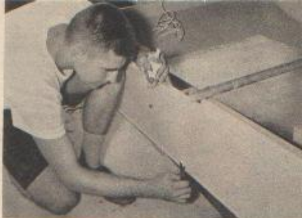
CALKING compound fills the recesses between sides and bottom reinforcing strips.
