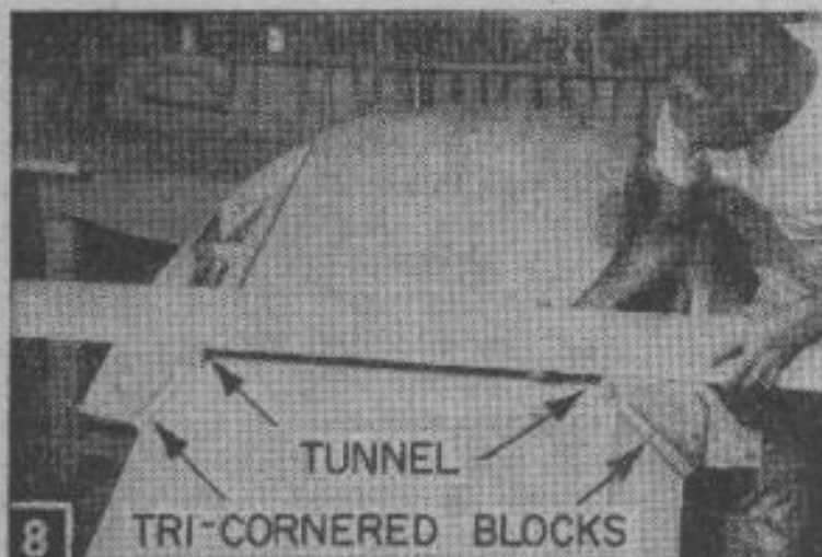
8 Aft end of fore plane bottoms must be in line and level, athwartships.
