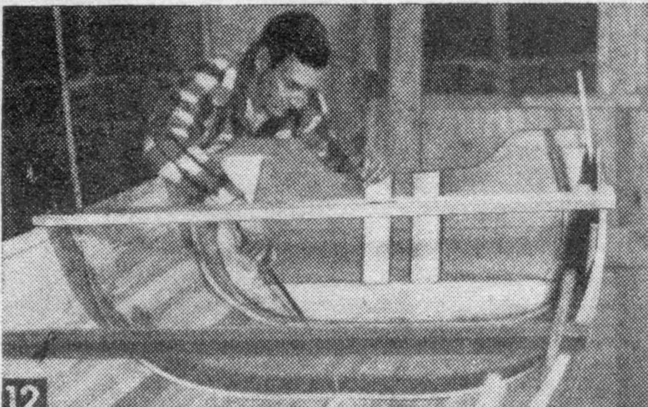
12 Frame positions are marked out by pencil with thin batten at 5 in. centers. Spring batten from sheer to sheer.
