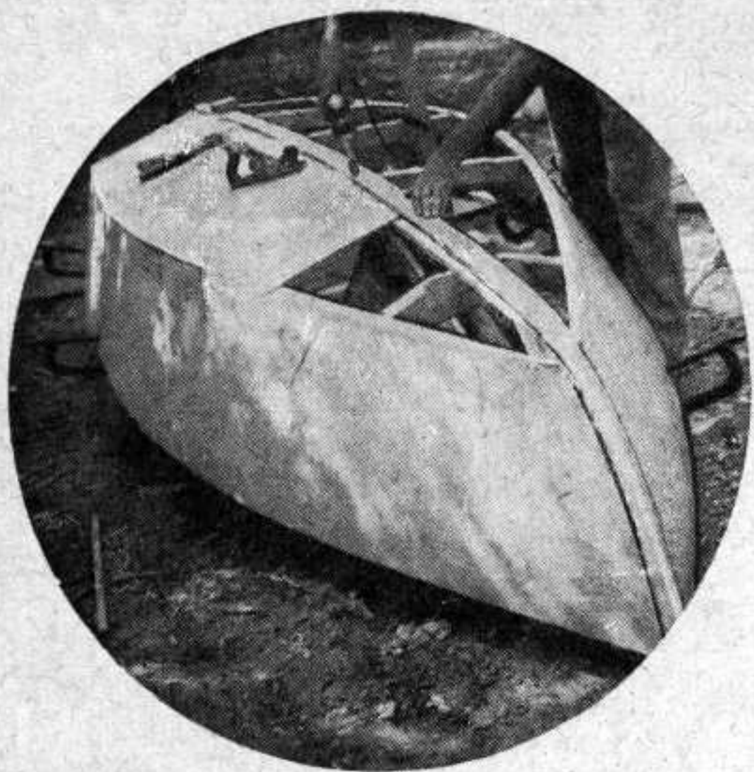
A small electric hand drill makes easier the work of planking the sides and bottom.
