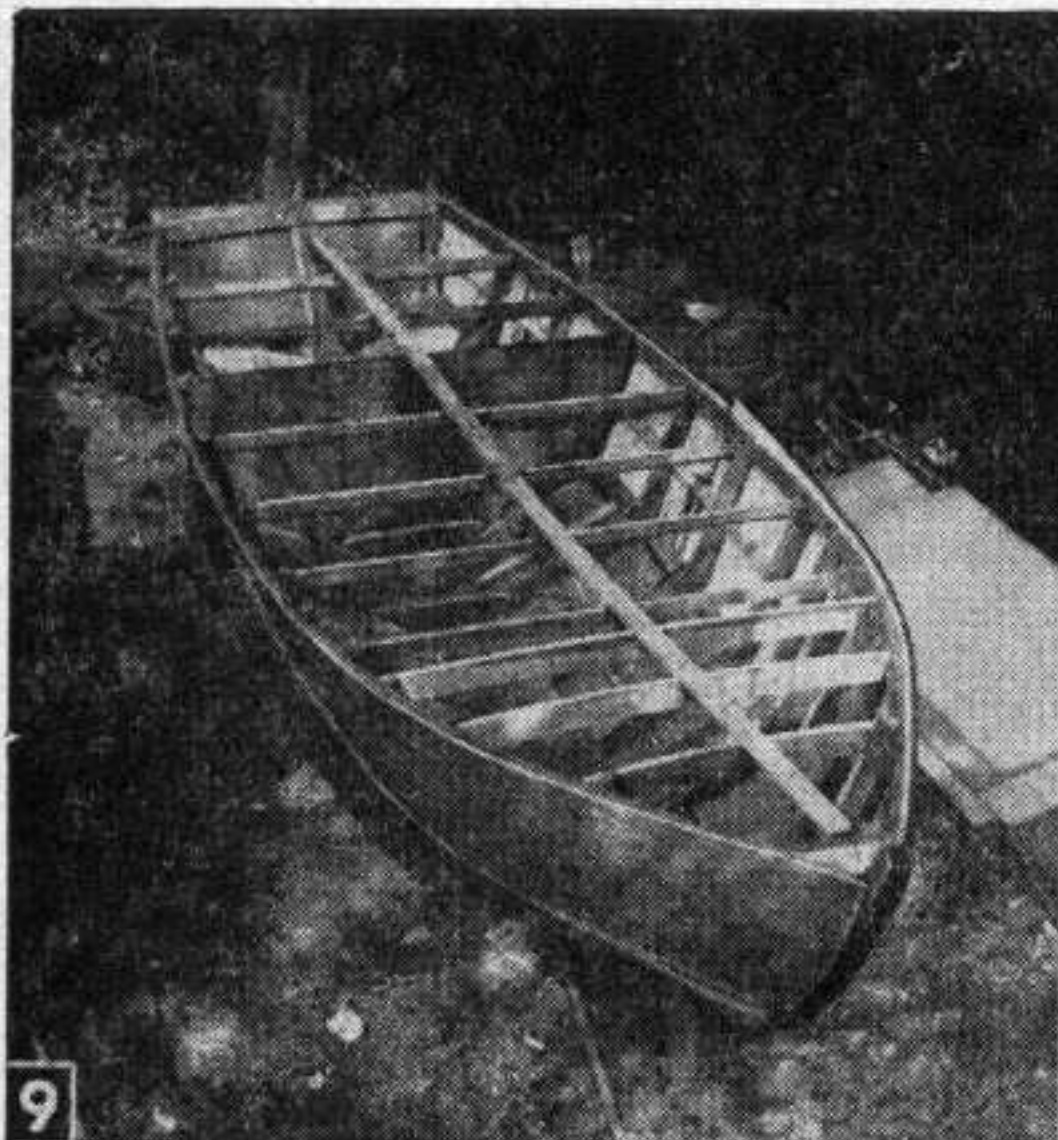
9 Deck beams are installed after planking is complete.
