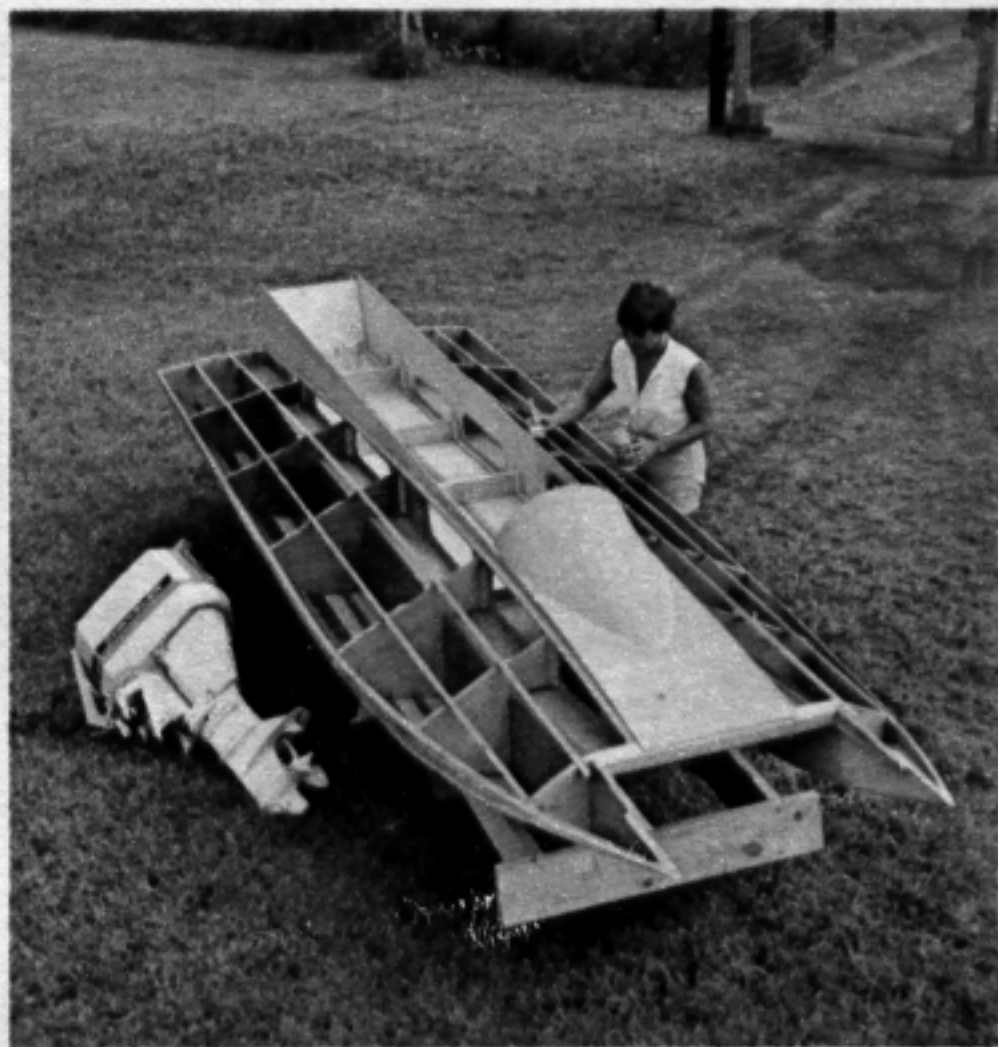
CRAFT is right side up on jig with several coats of varnish applied prior to decking.
